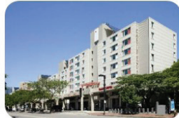
Castle Square, Boston MassHousing financed a deep energy retrofit of the 500-unit development, resulting in 50% reduction in energy usage.
