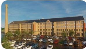
Stone Mill, Lawrence MassHousing financed the first all-electric mill conversion in MA, turning a vacant property into 86 units of affordable rental housing.
